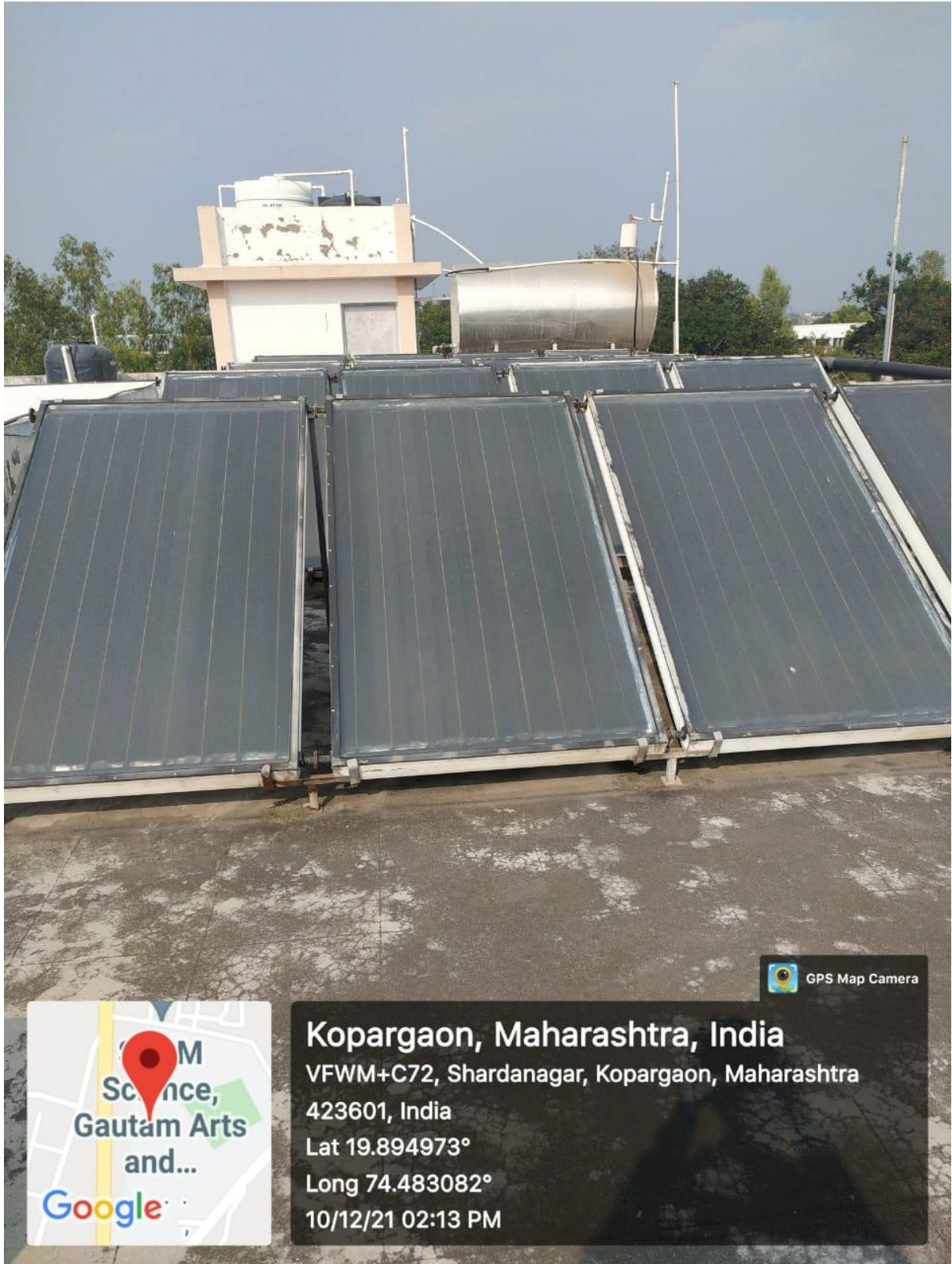
Panels of Solar Water Heaters
