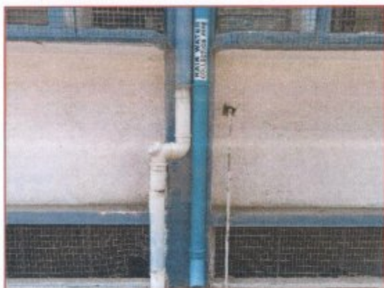
Rain Water Harvesting Installation unit (Work in progress)
