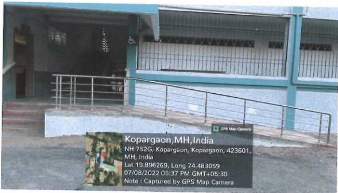
Ramp at 'A' Block
