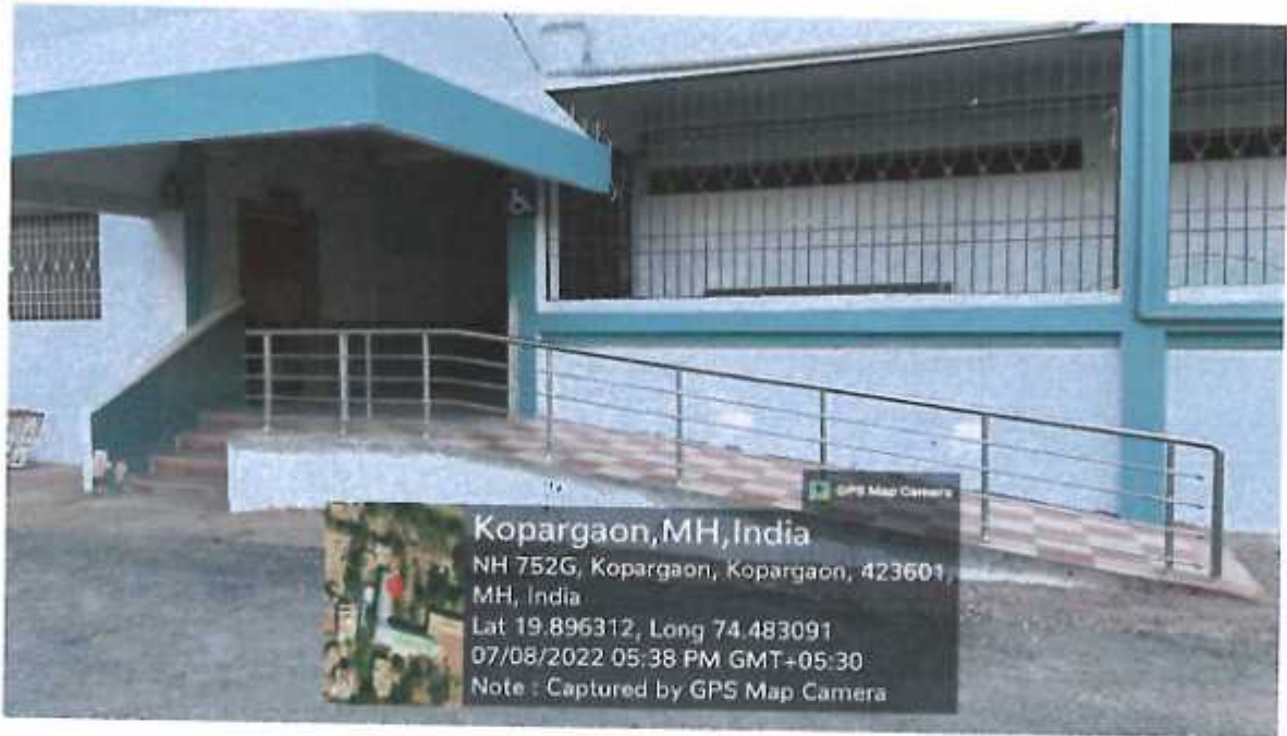
Ramp at 'A' Block
