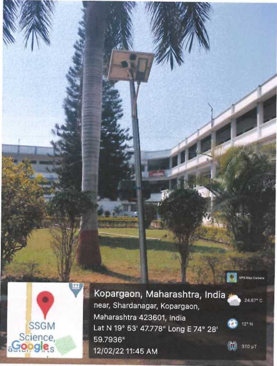
Sensor Based Solar Lights
