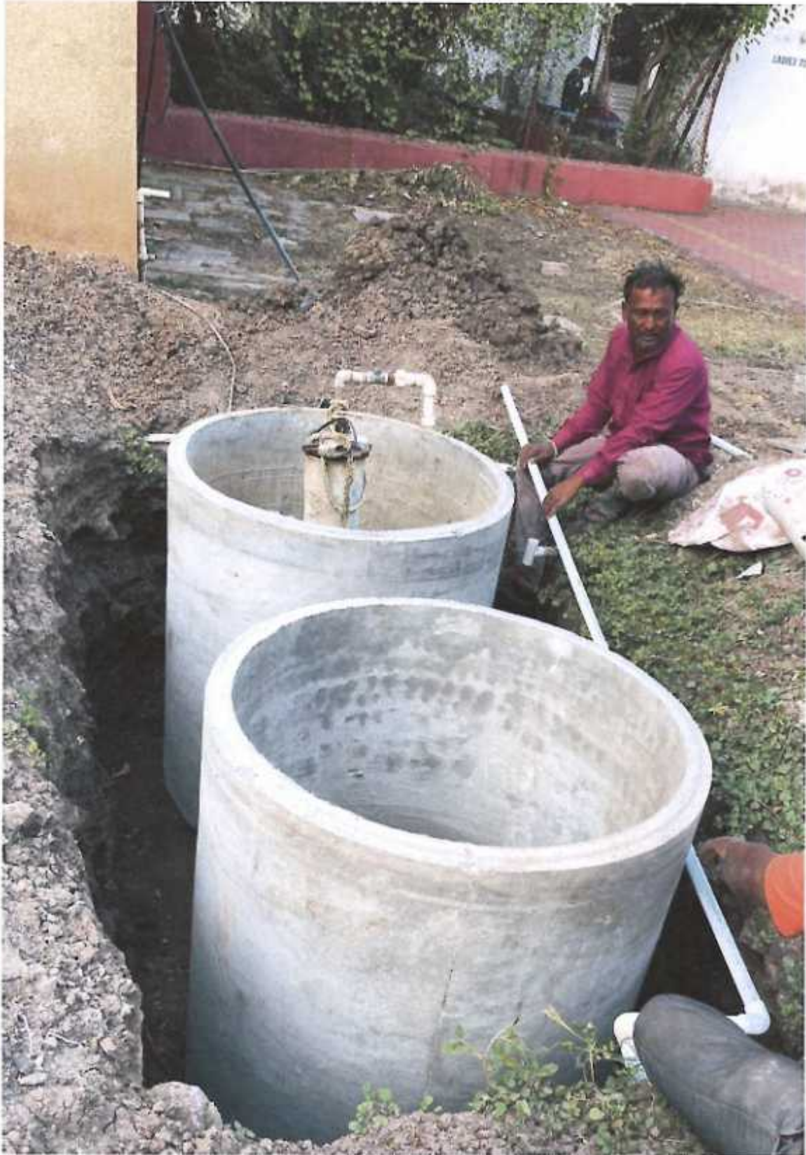
Bore well Recharge: work in progress
