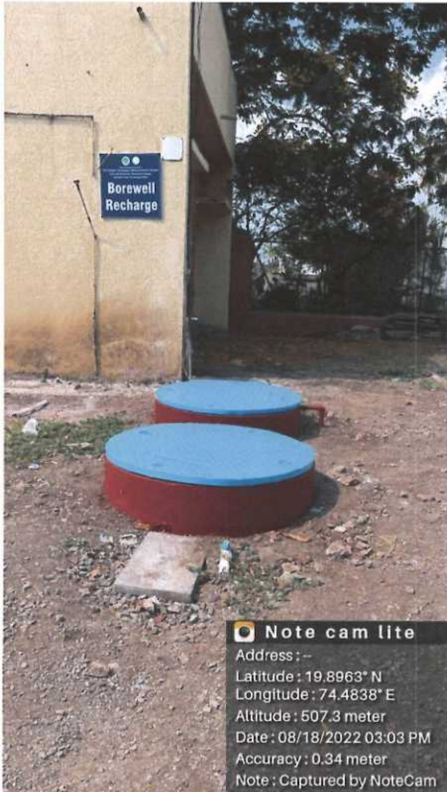
Bore well Recharge Facility
